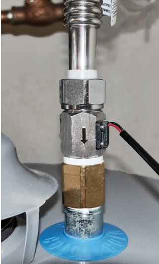
4. Disconnect the cold water supply line from water heater. Be careful not to bend and crease the supply line when manipulating it. Be prepared with some towels as some water will flow out of the hookup line. You don't have to drain the tank. As long as all the faucets remain closed you should not get any back flow from the hot water line.
