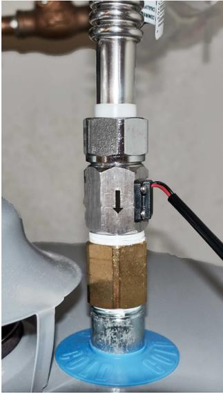
4. Disconnect the cold water supply line from water heater. Be careful not to bend and crease the supply line when manipulating it. Be prepared with some towels as some water will flow out of the hookup line. As long as all the faucets remain closed you should not get any back flow from the hot water line.
